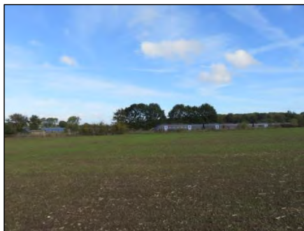
View north from footpath south of railway line showing solar farm in the distance.
